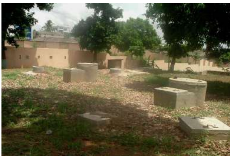
Biogas plant at the Accra Psychiatric Hospital
