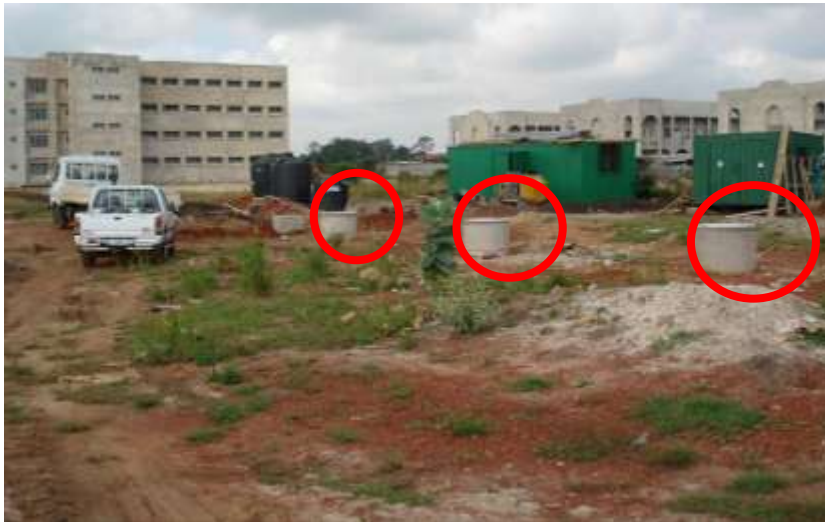
Three digesters built at the Central University College
