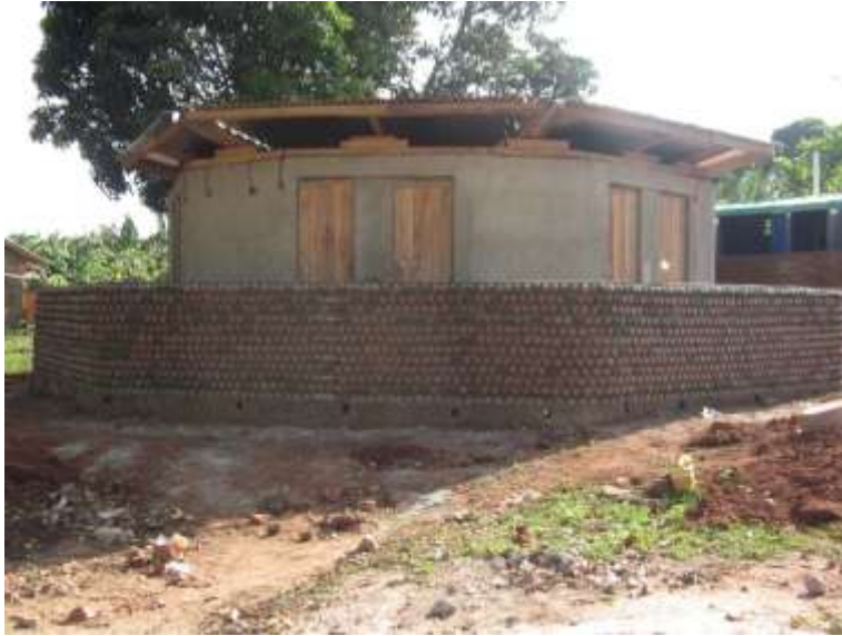
Completed institutional latrines which are connected to a biogas digester
