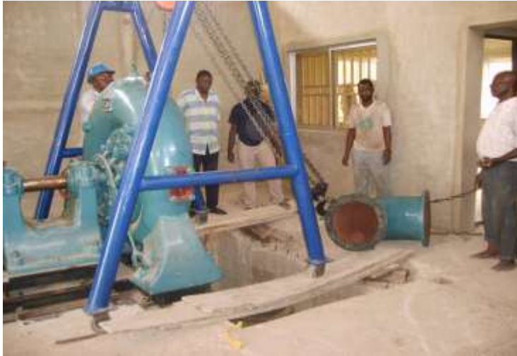
Installation of Turbines by Trainee Engineers and Technicians
