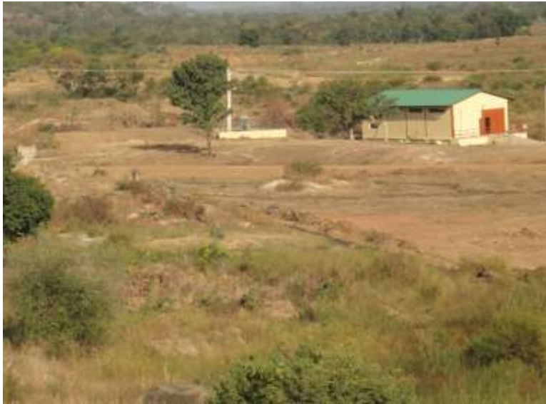
Completed Waya Project Showing Power House and Transformer
