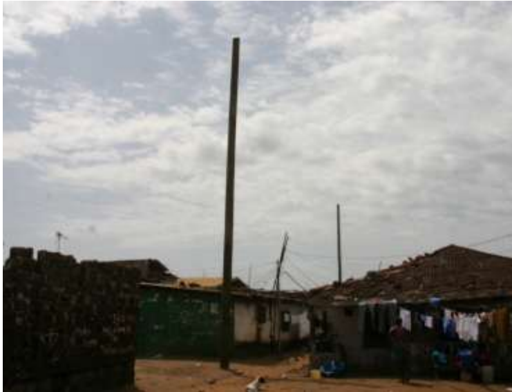
Illegal connections prevalent in informal settlements before Liberia Electricity Corporation began electrifying the residents
