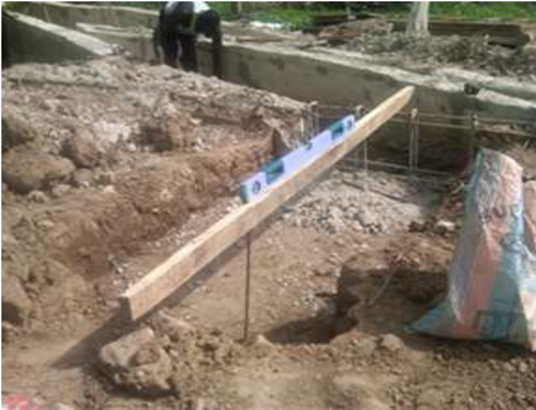
Setting out of the power house floor
