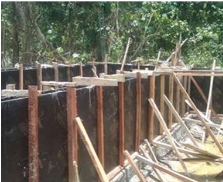
Form work for tailrace canal
