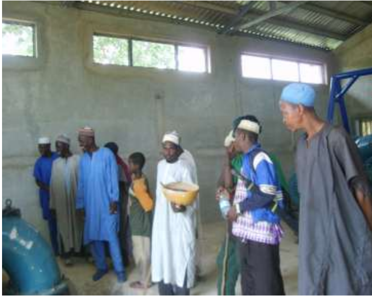
The Community During the Equipment Installation Process
