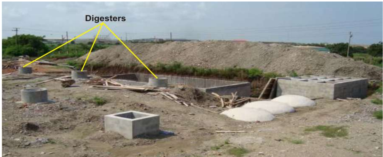
Digesters under construction
